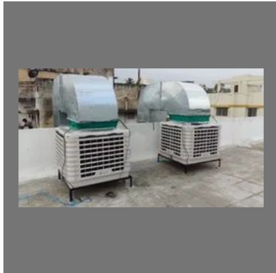
Air Ducting Installation Services
