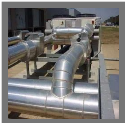
Insulation Duct Pipe Installation Service
